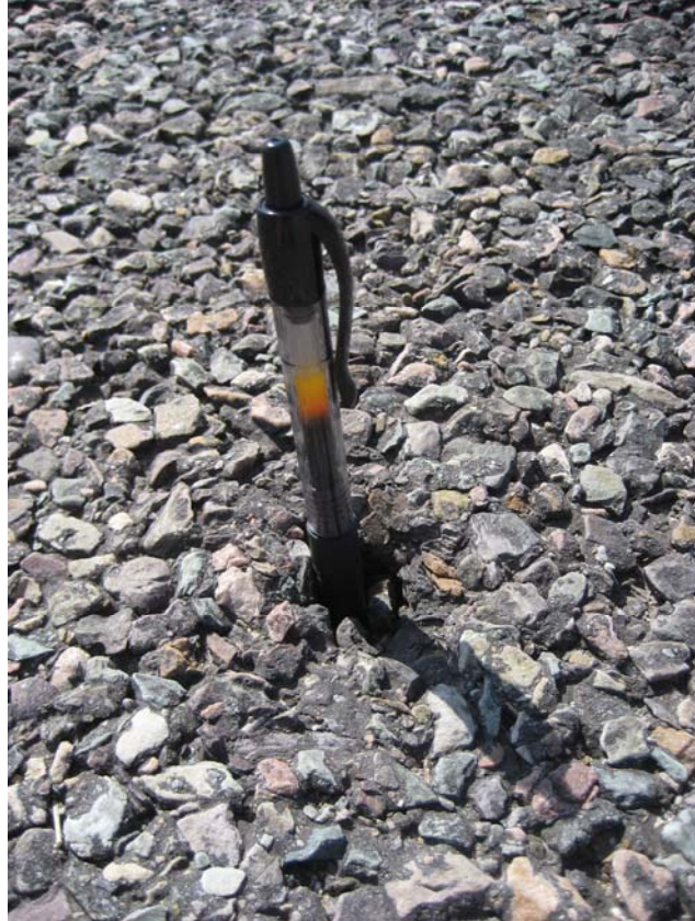
Image: 1.3.2.2 PFC Popout on Taxiway A
