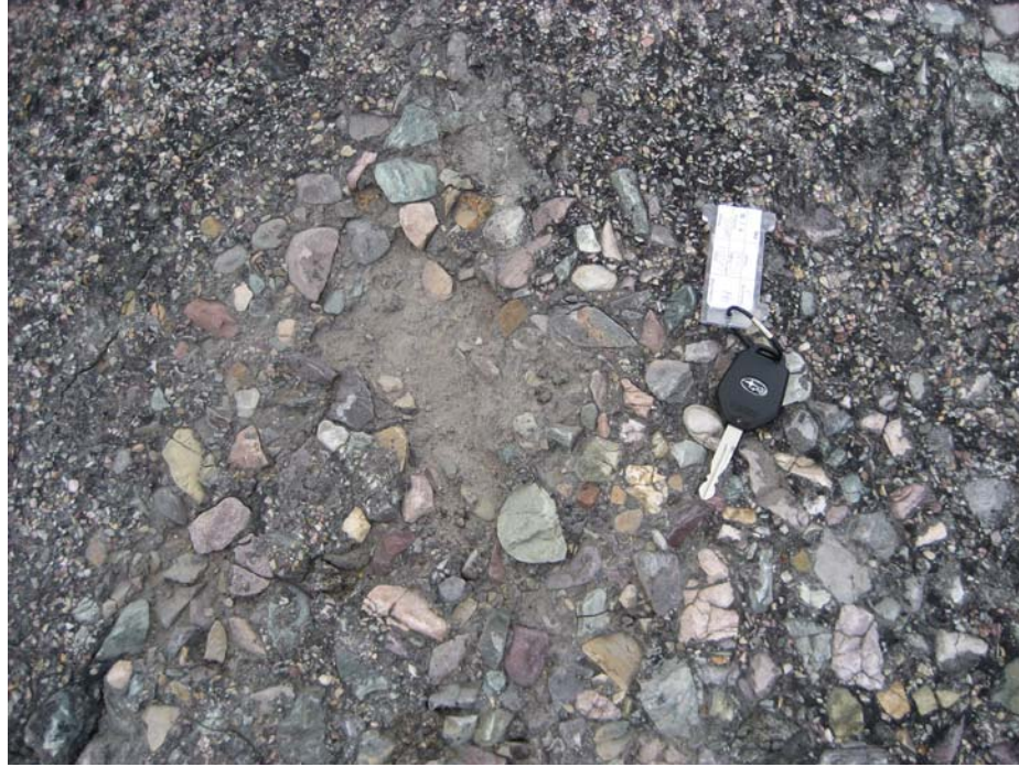
Image 1.3.2.3 High Severity Weathering on Taxiway E
