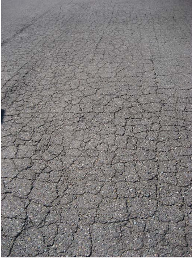
1.3.3.2 Medium Severity Alligator Cracking on the Airborne Apron
