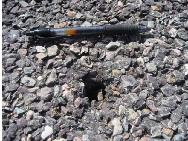
Image: 1.3.2.1 PFC Popout on Taxiway A
