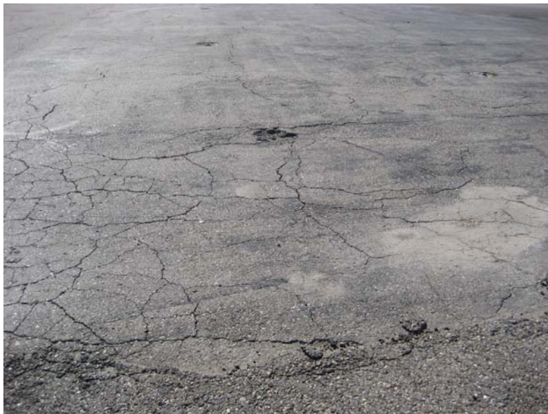
1.3.3.3 Medium Severity Alligator Cracking and High Severity Raveling causing Excessive FOD on the Airborne Apron
