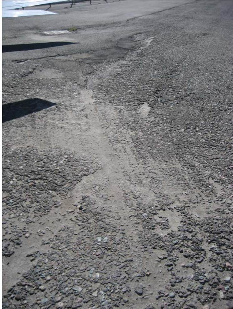
Image 1.3.3.1 High Severity Weathering on General Aviation Apron-West (GA-West4)
