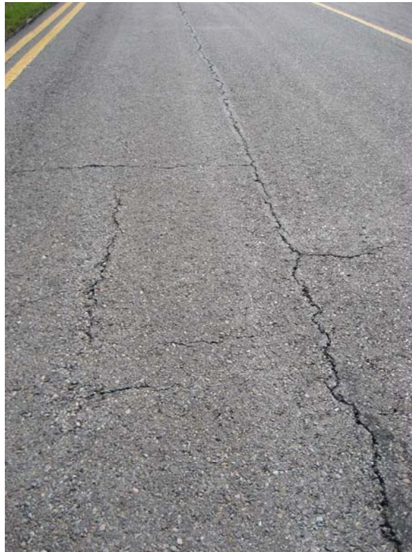
Image 1.3.2.5 Block Cracking on the Southern Portion of Taxiway G
