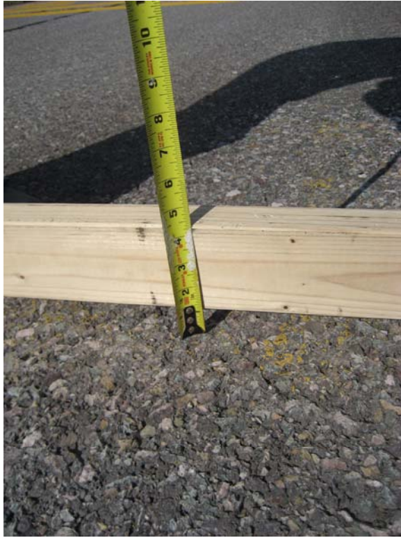
Image 1.3.2.4 Medium Severity (1" depth) Depression on the Northern Portion of Taxiway G
