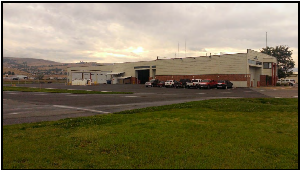
SRE/ARFF Equipment Storage Building
