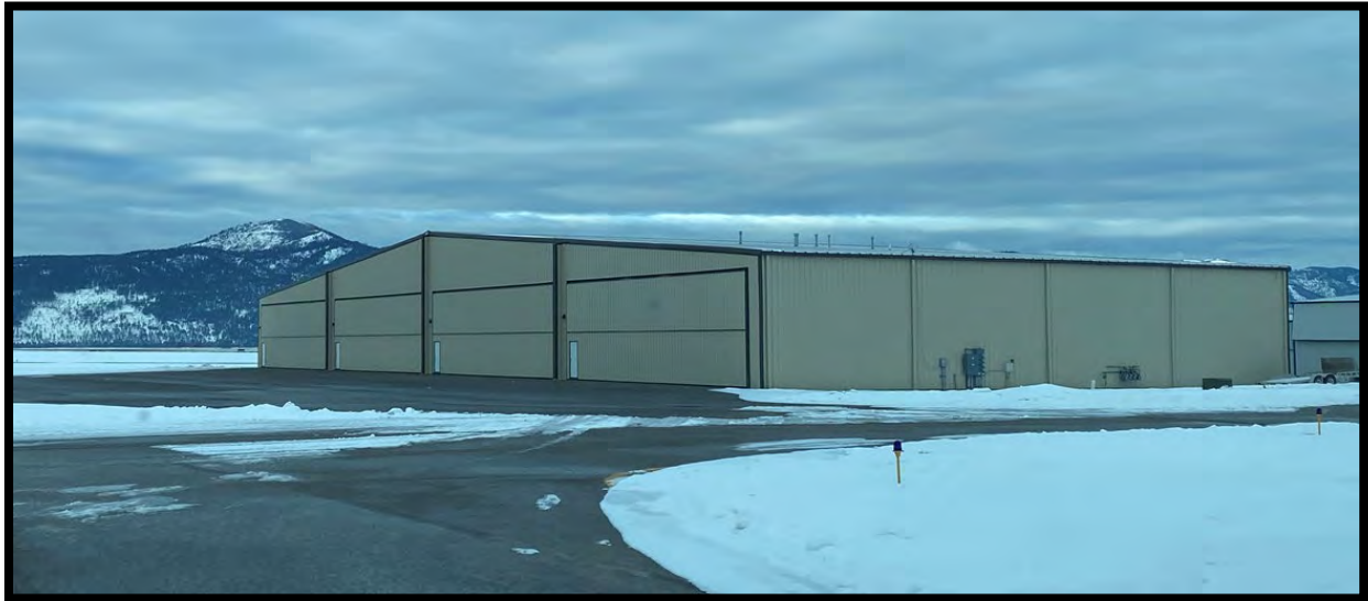
Delta Hangar – West of Deicing Apron
