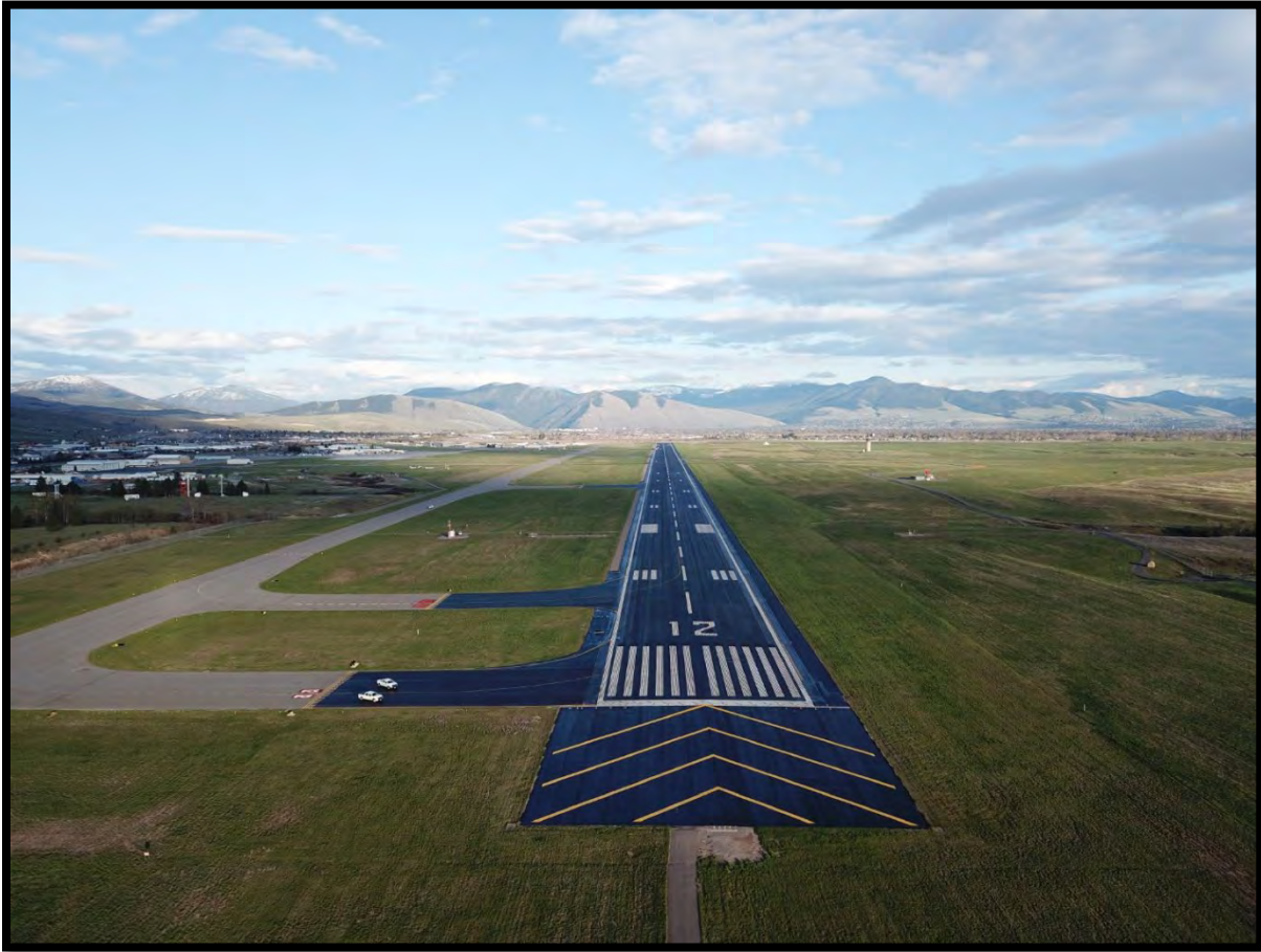
Newly rehabilitated Runway 12-30 in 2018
