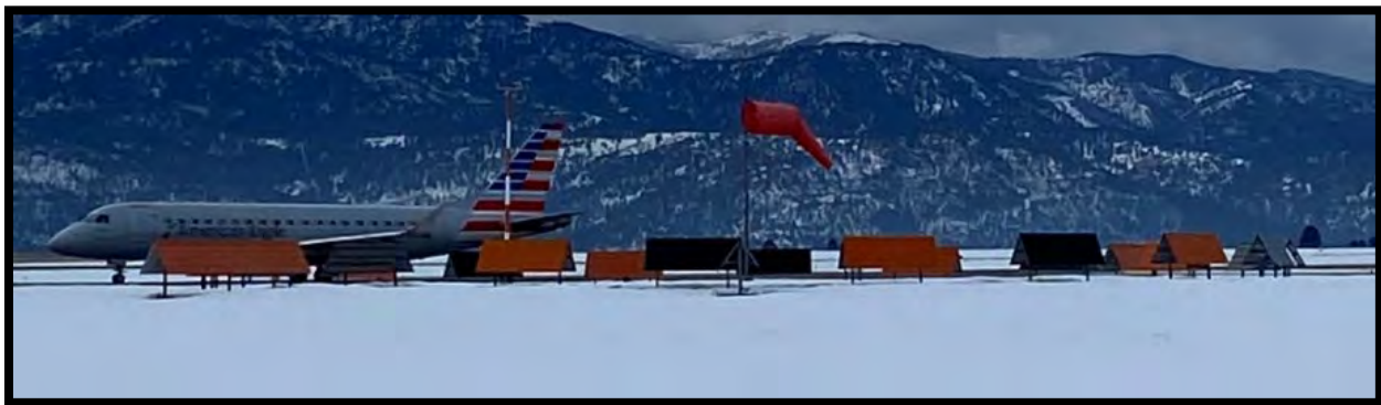
SEGMENTED CIRCLE AND WINDCONE
