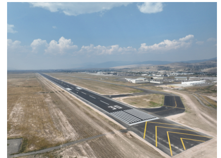
Massive runway rehabilitation project completed Read more
